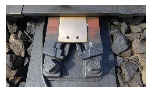
The Lube EP backpack application method is quicker than the conventional brush method, safer, and more precise. It will not impact the environment due to the low application quantities, 4ml per chair and 95% biodegradable credentials.
